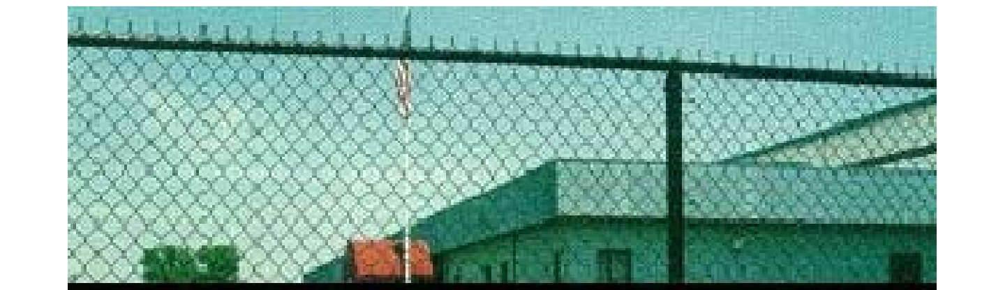
ALL FENCE TO BE 6' BLACK POLYVINYL CHAIN LINK NOT TO SCALE
