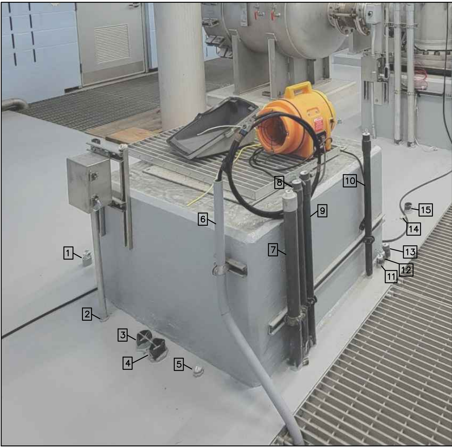
PHOTO 1 – EXISTING HPP-9 CONDUIT STUBS NOT TO SCALE
