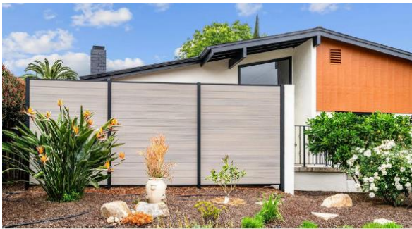
WPC River Birch composite fence installed adjacent to residence — shows natural wood-grain finish, horizontal board orientation, and black aluminum post-to-panel connection
