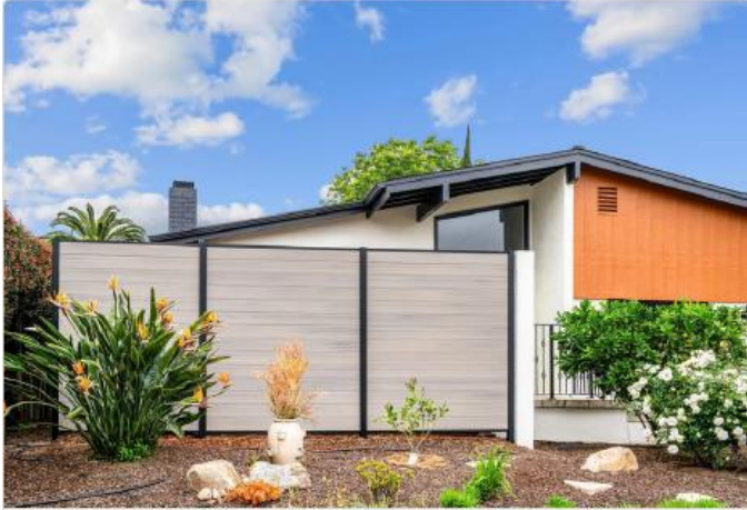
WPC River Birch composite fence installed adjacent to residence — shows natural wood-grain finish, horizontal board orientation, and black aluminum post-to-panel connection
