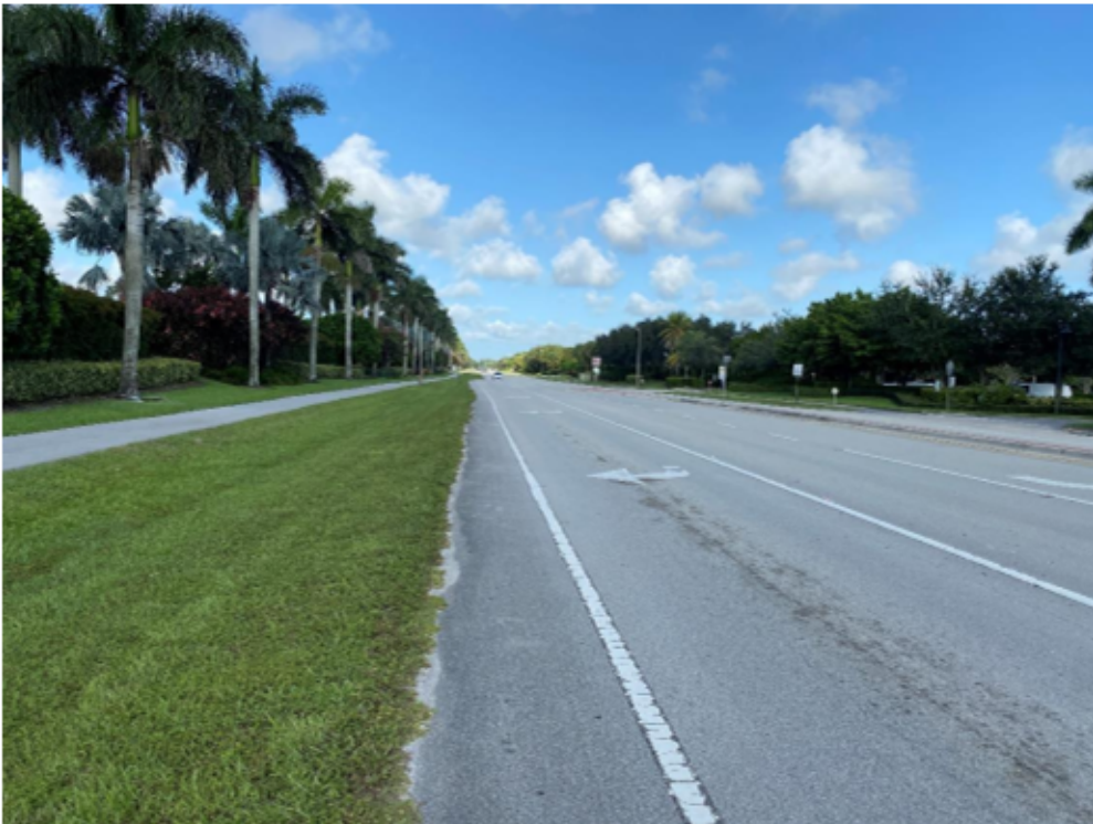
LOOKING WEST ALONG STRIBLING WAY WITH SUBJECT AT LEFT
