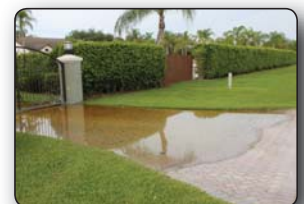
The Absence of Swales or Appropriate Culverts Results in Ponding
