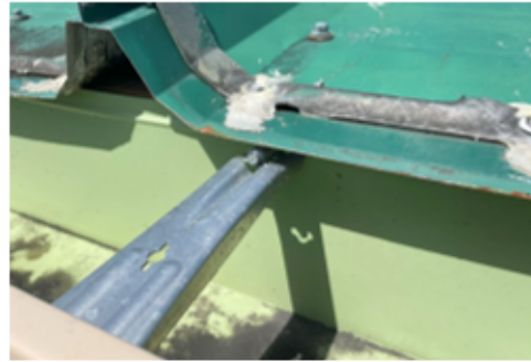
Gutter bracket thru drip edge
