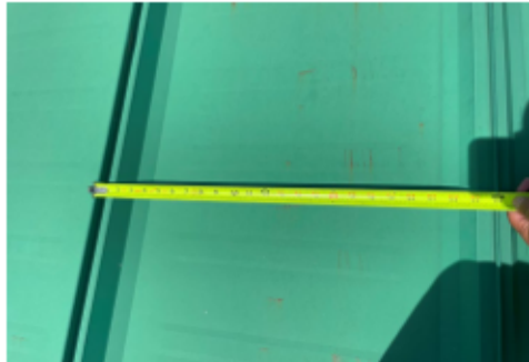
Metal roof profile 24" rise to rise
