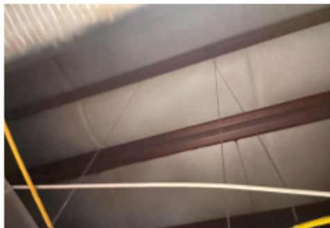
Beams and insulation
