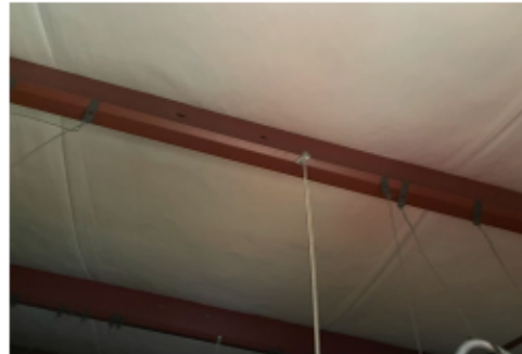
Beams and insulation
