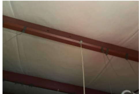
Beams and insulation
