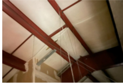
Beams and insulation
