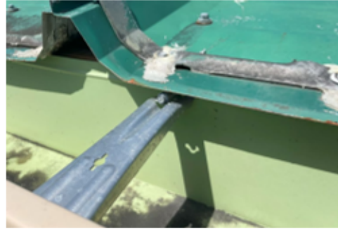
Gutter bracket thru drip edge
