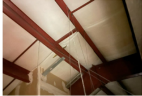
Beams and insulation
