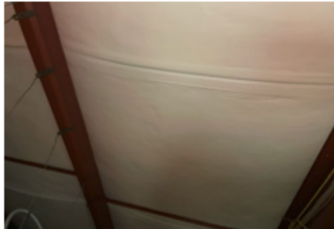
Beams and insulation
