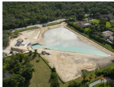
Deering Estate Flow-Way Pump Station (S-700)
