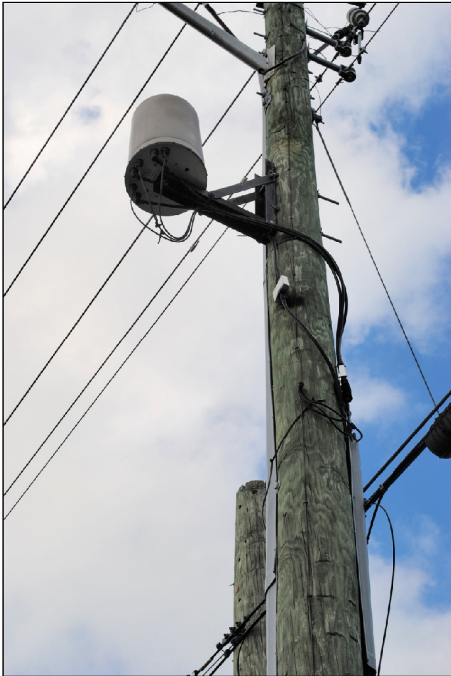
Figure 12. A close-up of one of the DAS antennas. Carrier objections to using this technology might include additional expense of obtaining rights-of-way, equipment costs, installation complexity and maintenance retraining.
