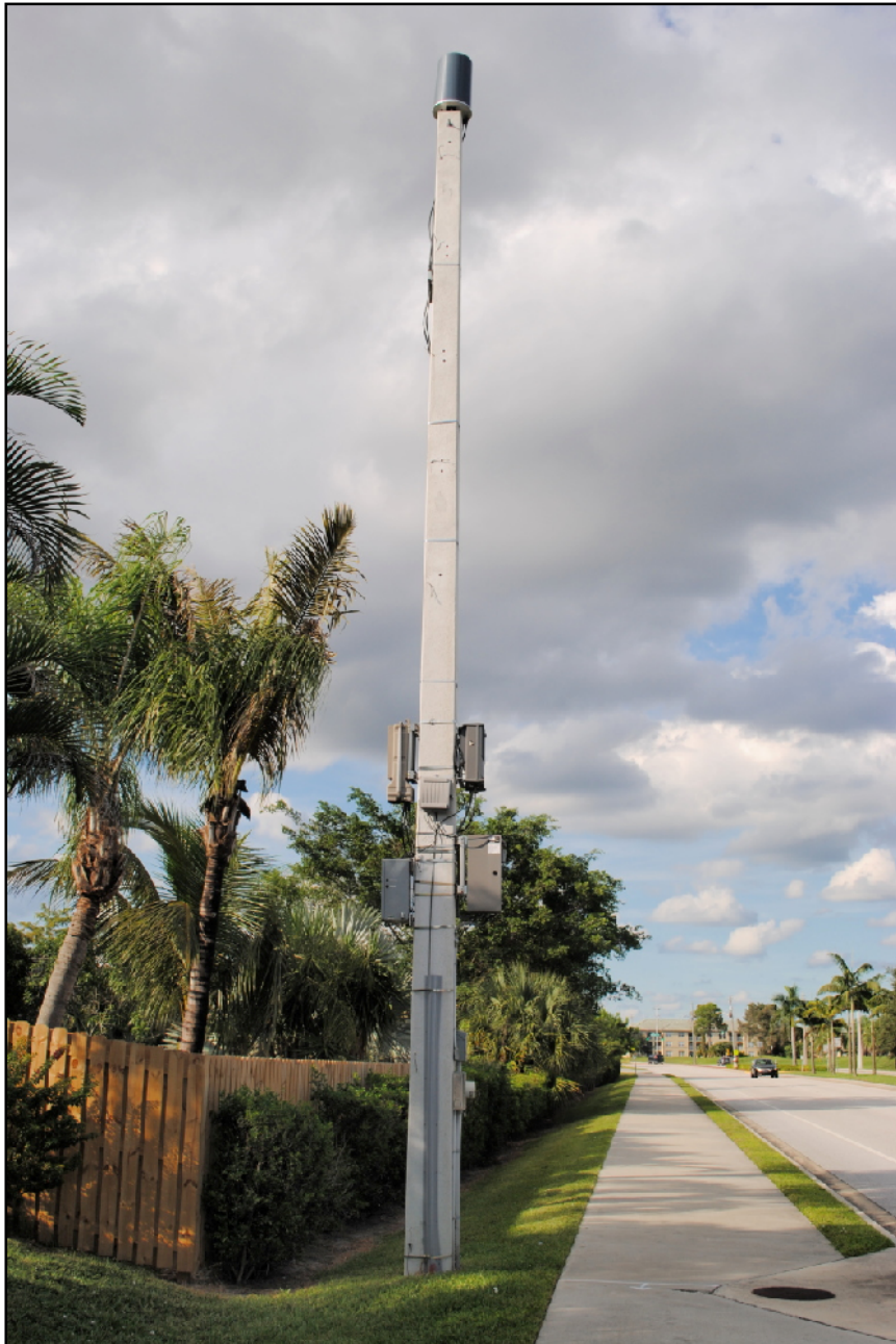
Figure 11. Distributed Antenna System (DAS) node location near the intersection of Carlton St. and Greenview Shores Blvd. This technology allows the “head-end” base station compound to be located at an inconspicuous place up to several miles from the neighborhood. The radio signals between antenna location and base station are transmitted as light along fiber optic cable to small cell installations such as this one. This is a mature technology and is available to all carriers.
