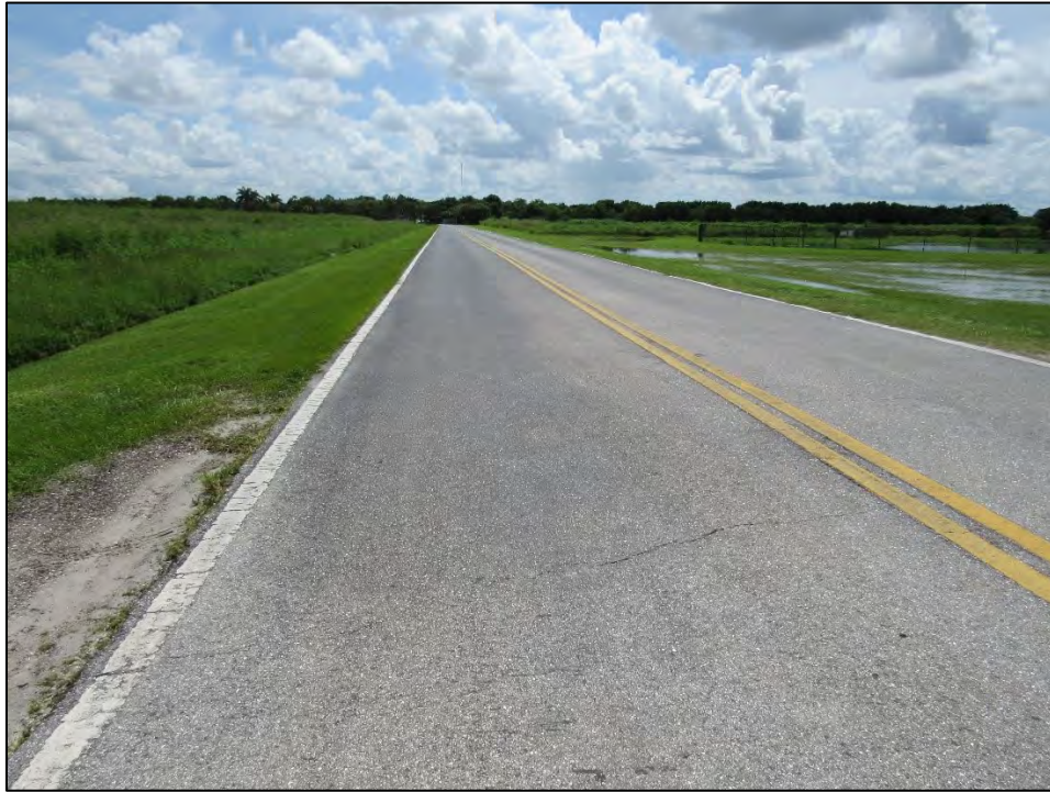
View looking south along temporary driveway easement with the subject on both sides
