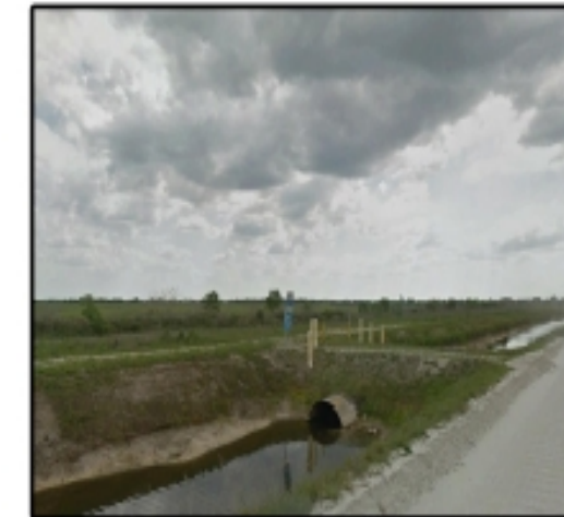
CROSSING ONTO ORANGE TRAIL
