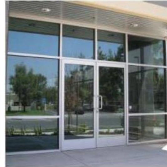
ALUMINUM STOREFRONT SYSTEM IN MANUFACTURER STANDARD CLEAR ANODIZED ALUMINUM FRAME WITH LIGHT GRAY TINTED GLASS
