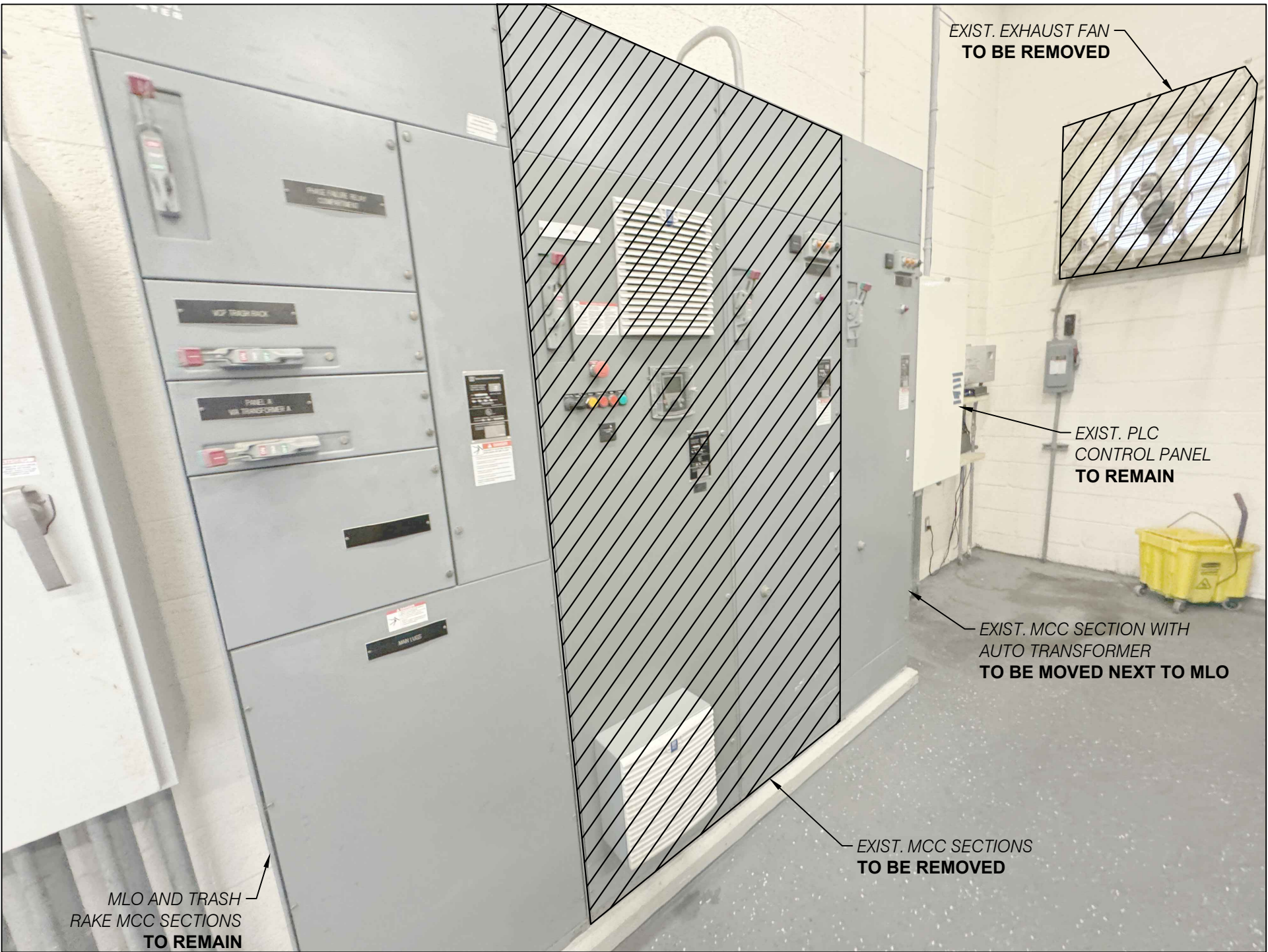
8 P7-C2 SITE PHOTO FACING EAST NTS
