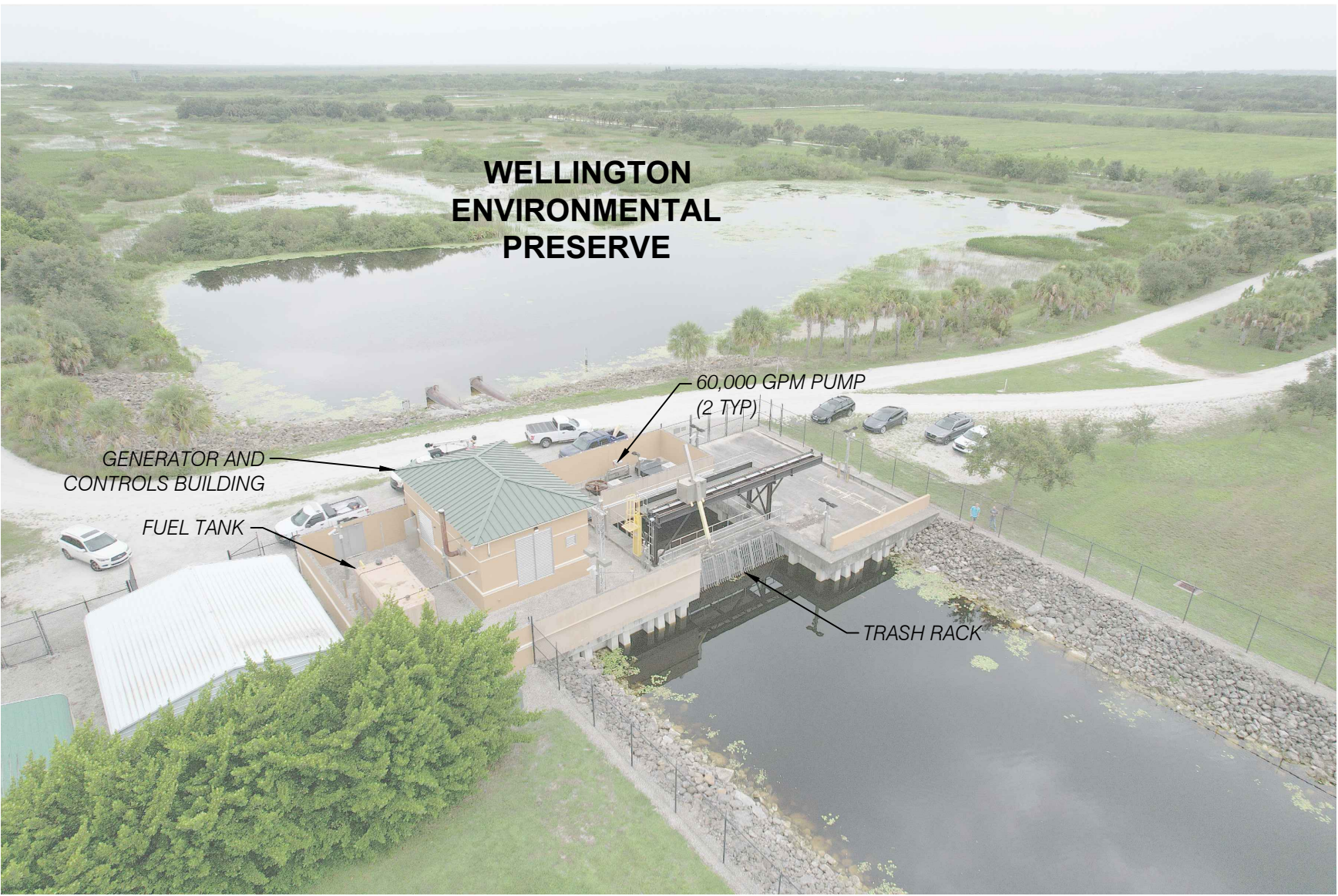
1 AERIAL PHOTO FACING NORTH EAST P9-C1 NTS
