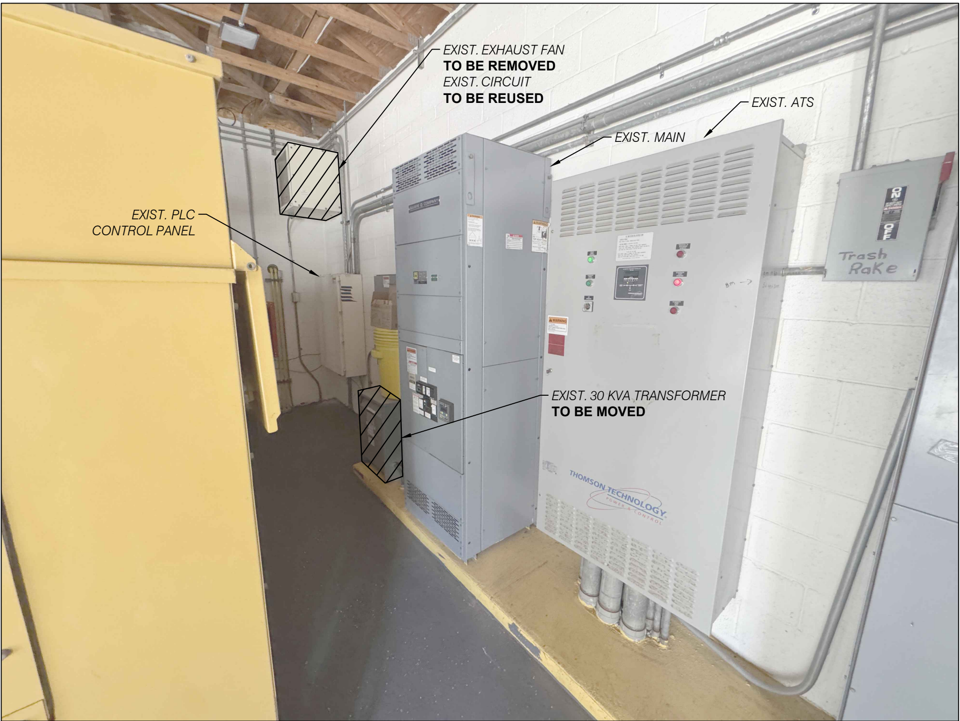
8 SITE PHOTO FACING SOUTH WEST P6-C2 NTS
