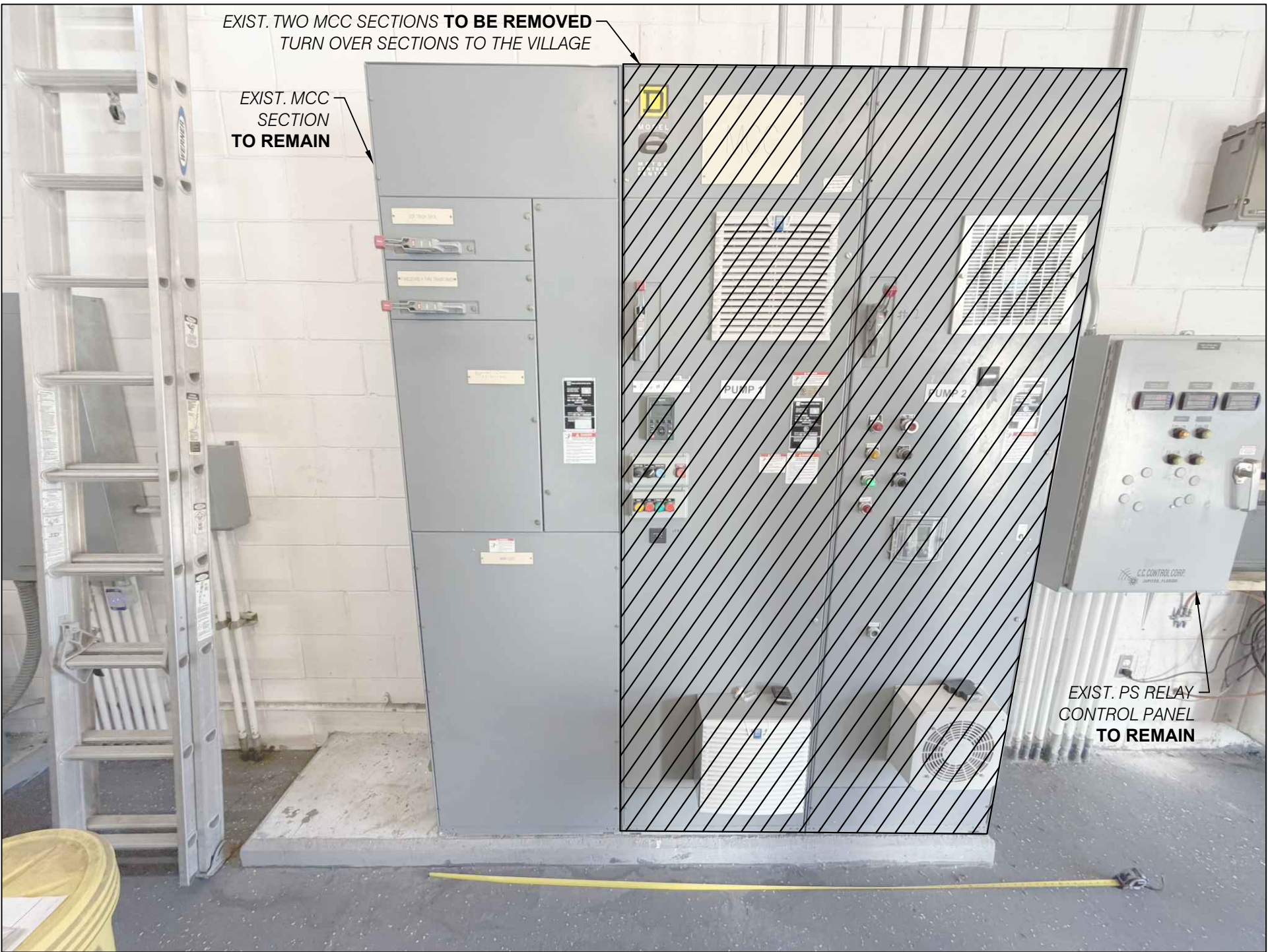
8 SITE PHOTO FACING WEST P8-C3 NTS
