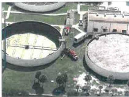
Clarifier pressure pipe rehabilitation at WWTP
