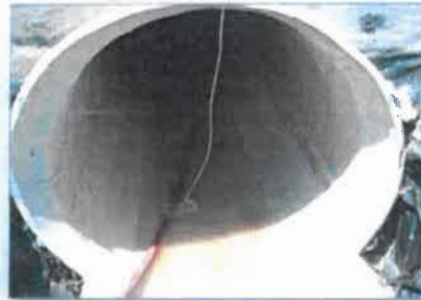
Finished outfall product at the headwall
