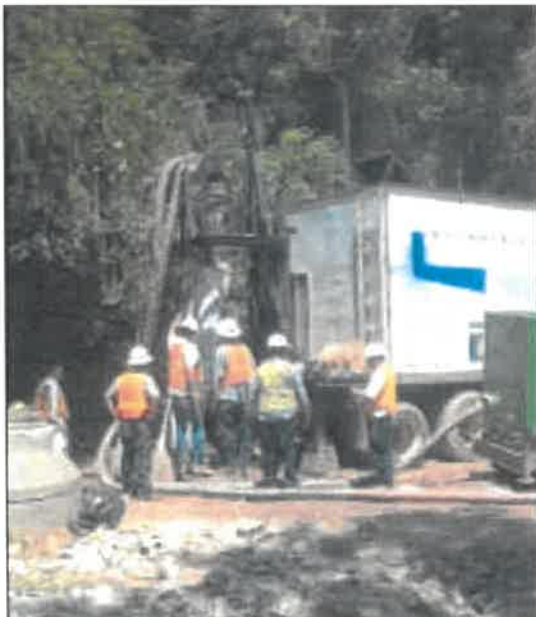
Easement installation of subdivision sewer rehab
