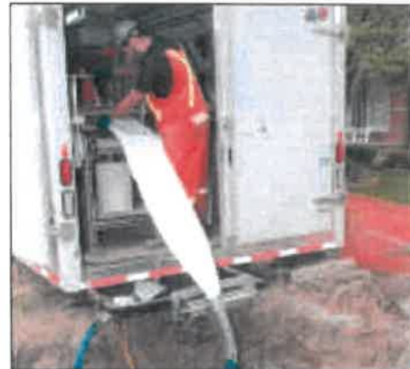
ASTM F1743 Pull & Invert technology
