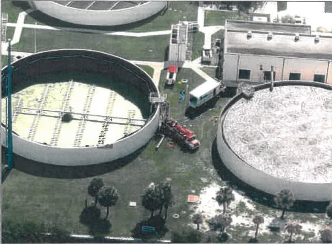
Clarifier pressure pipe rehabilitation at WWTP
