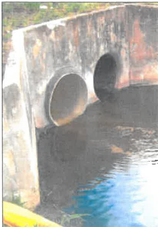
Trenchless renovation in storm drain application
