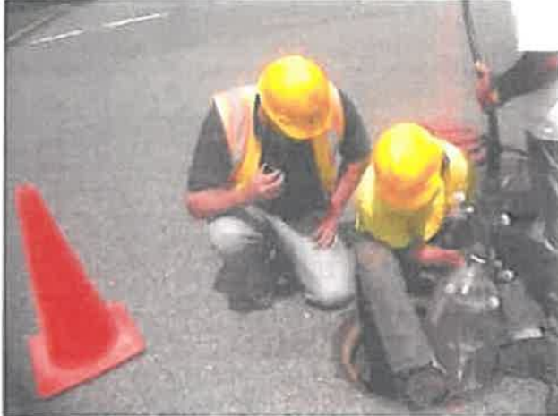
(Figure #3 Light Train inserted into a 30" Trunk Sewer on Division Street)
