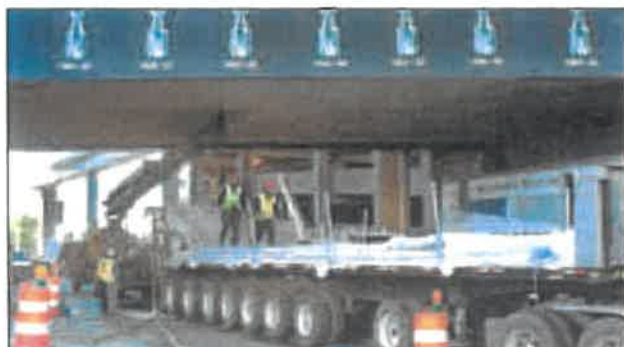
Large bore trenchless renovation in "tight quarters"
