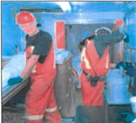
NSF 61 Certified water main rehabilitation
