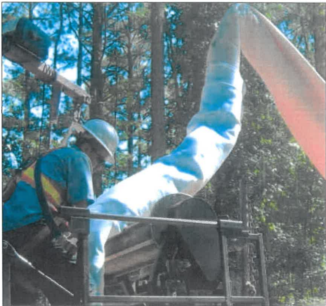
Lanzo Lining Services crew preparing liner for direct inversion installation of CIPP
