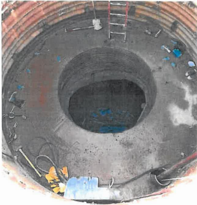
As part of the Segment 4 repairs, a suite of trenchless methods were used, including CIPP, cementitious Centripipe and grout-in-place liners.
