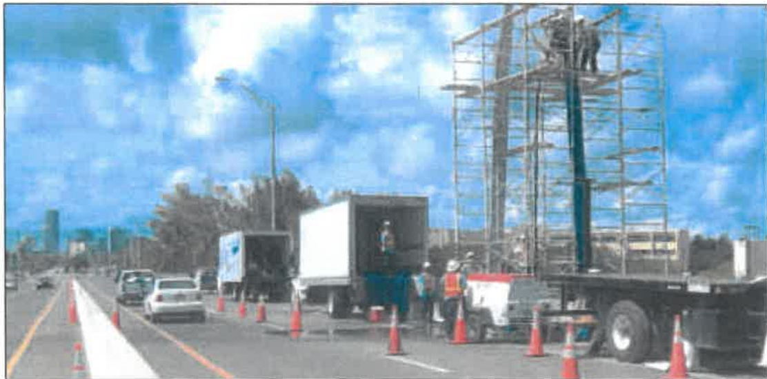
Trenchless CIPP rehabilitation of a pipe running under a busy highway during rush hour traffic
