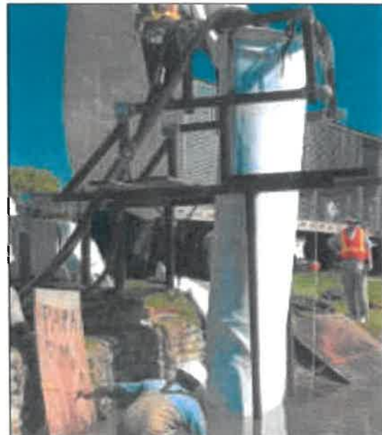
Subaqueous installation of CIPP into storm drain
