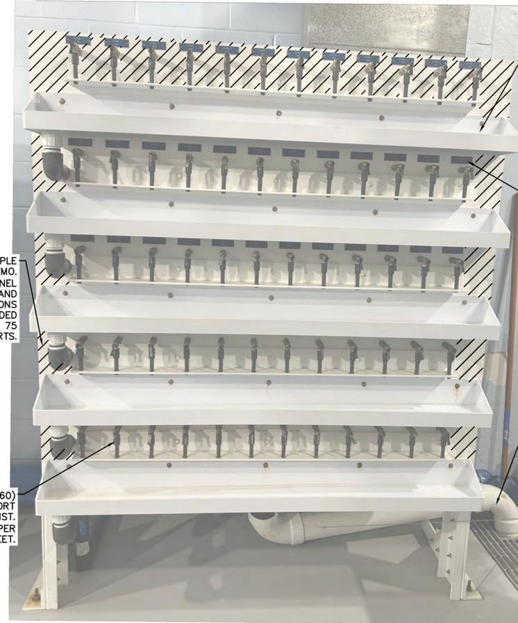
REMOVE EXIST. SAMPLE PORTS AND DEMO. EXIST. 61.5"x60" PANEL. CONST. NEW PANEL AND ADD PENETRATIONS AS NEEDED TO ACCOMMODATE 75 SAMPLE PORTS.
