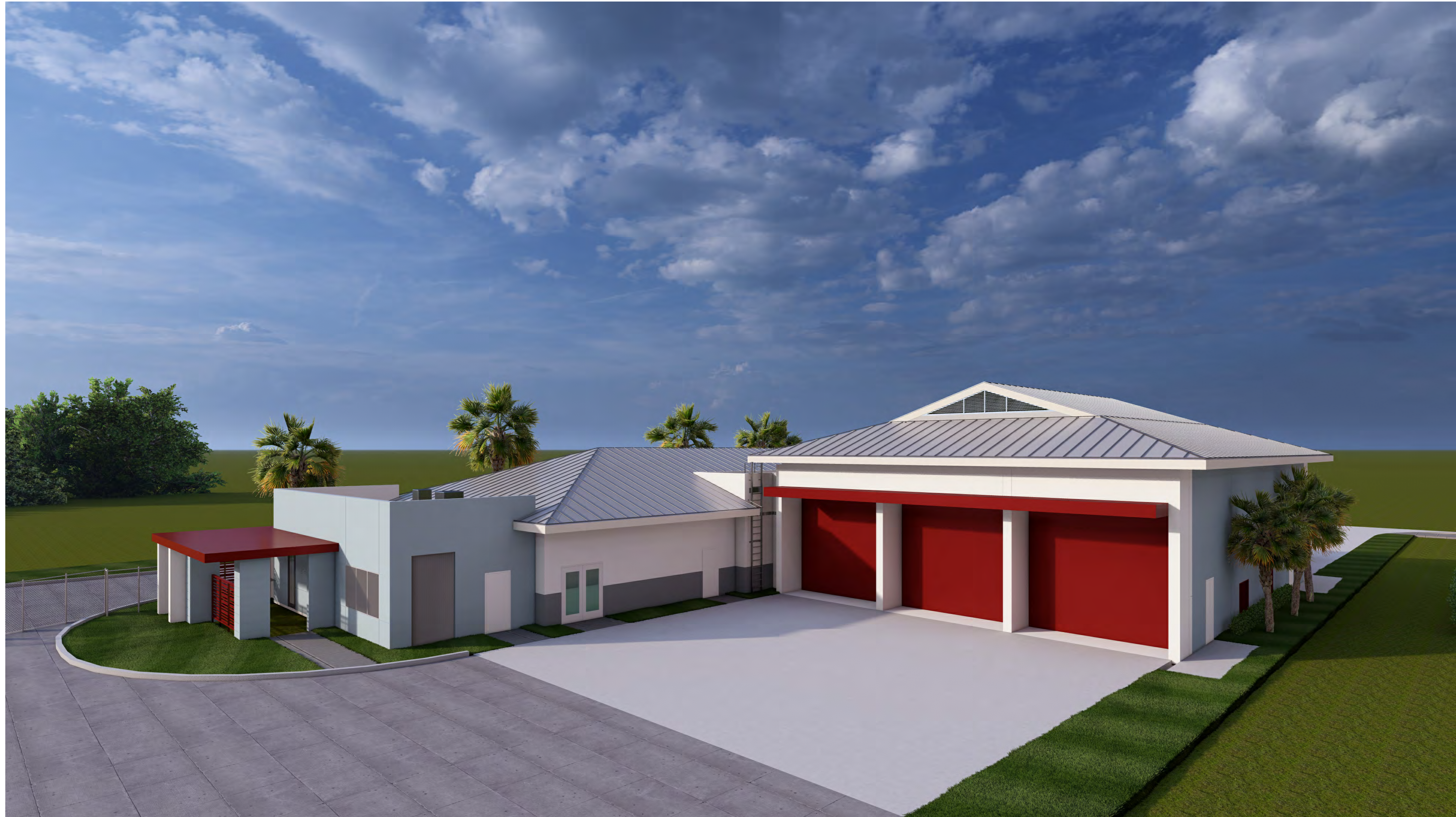
PALM BEACH COUNTY FIRE RESCUE STATION 25
