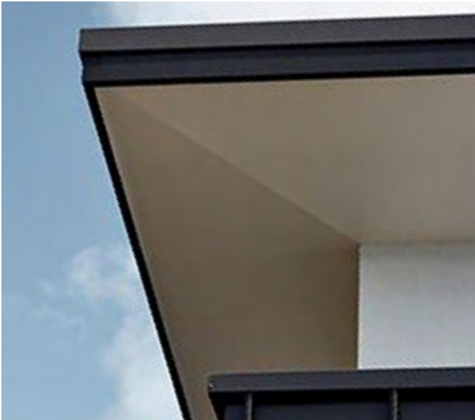
FASCIA AND SOFFIT
