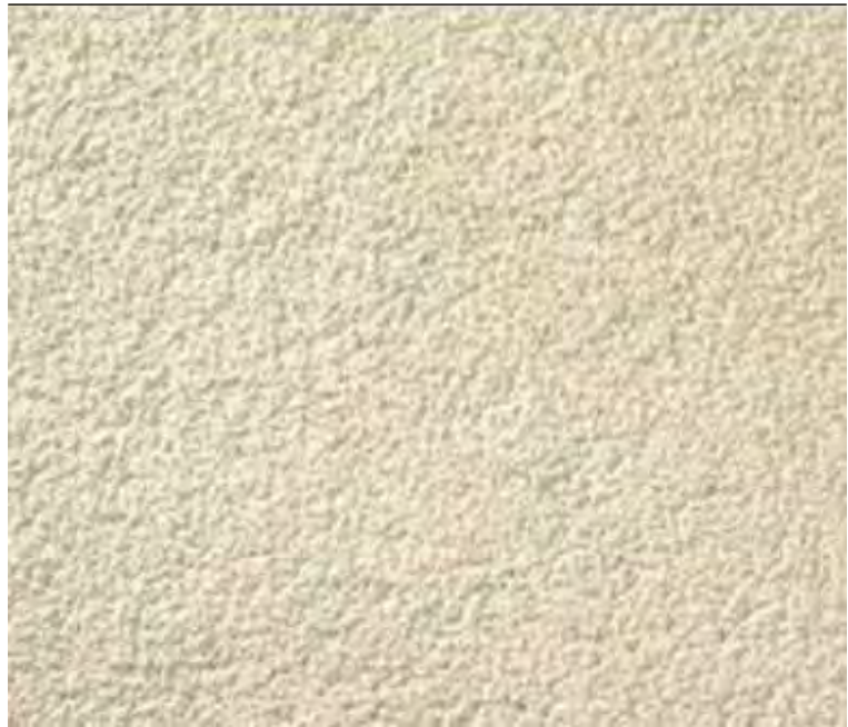
3 COAT STUCCO VENEER LACE FINISH W/ VERTICAL AND HORIZONTAL SCORING
