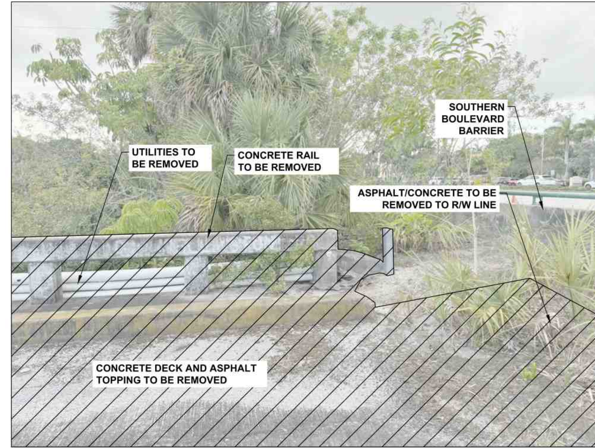
6 SITE PHOTO - FACING NORTHWEST C1-3 NTS
