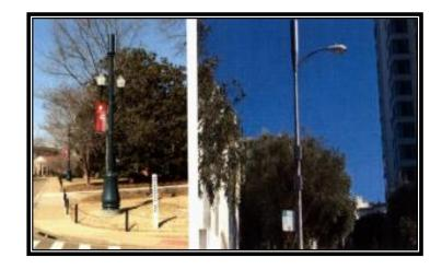
All collocations on existing utility poles shall utilize shrouds or canisters to conceal the antenna mounted on the top of the utility poles, such as the examples below, and shall either route transmission lines and cables through the interior of the poles when possible or use color matched conduit to conceal lines and cables on the exterior of the existing poles:
