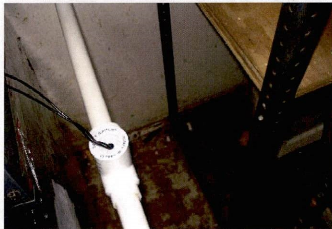
Drain line not insulated or supported FBC 5th Edition Mechanical 307.2.5
