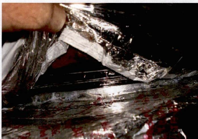
Flex duct not installed properly FBC 5th Edition Mechanical 603.9/Residential M1601.4.2
