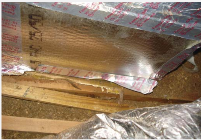
Return air not sealed properly FBC 5th Edition Mechanical 603.9
