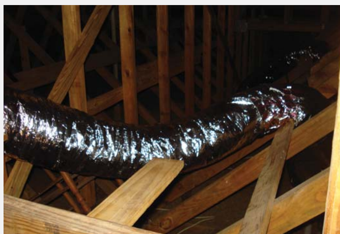
Flex duct not supported properly FBC 5th Edition Mechanical 603.10
