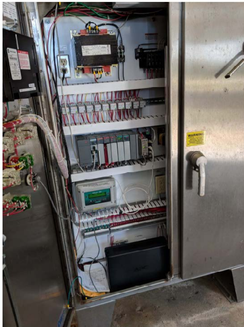
Seepex Control Panel PLC (Cake Pump)
