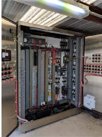
Gravity Filter MCP Enclosure
