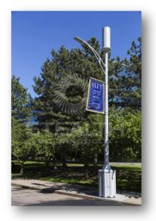
All collocations on existing utility poles shall utilize shrouds or canisters to conceal the antenna mounted on the top of the utility poles, such as the examples below, and shall either route transmission lines and cables through the interior of the poles when possible or use color matched conduit to conceal lines and cables on the exterior of the existing poles:
