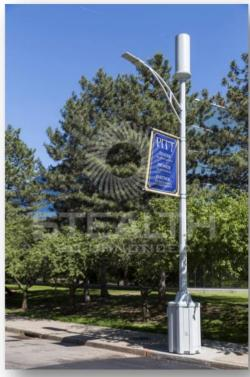
All collocations on existing utility poles shall utilize shrouds or canisters to conceal the antenna mounted on the top of the utility poles, such as the examples below, and shall either route transmission lines and cables through the interior of the poles when possible or use color matched conduit to conceal lines and cables on the exterior of the existing poles:
